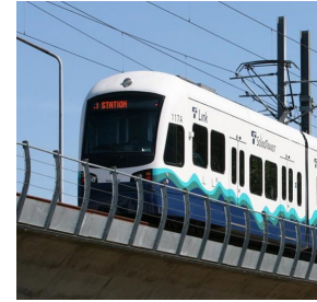
ST Link Light Rail
